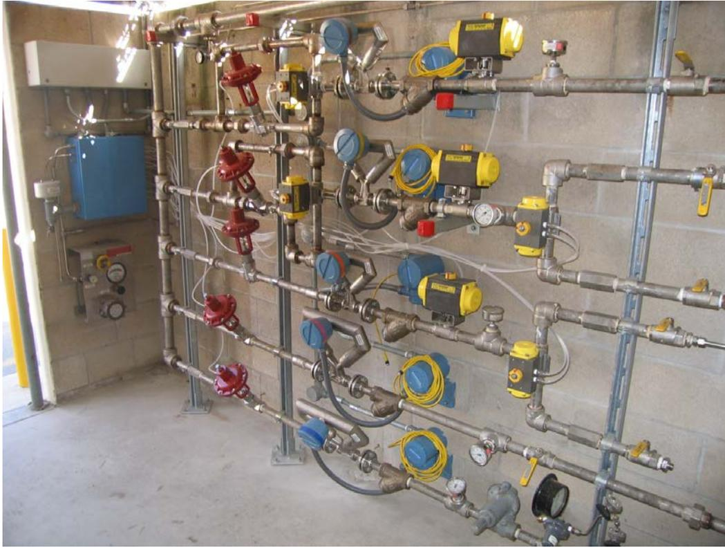
**Figure 15. Gas Mixing Station.**
